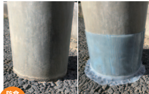
防食 Anti-corrosion 管柱地際の防食 Corrosion protection at the pipe column bases
