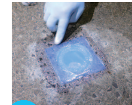
止水 Water stop 鉄道穴塞ぎ Railway hole blockage
