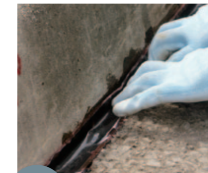
その他 Other 道路と縁石間の植生防止 Prevention of vegetation between the road and the curb
