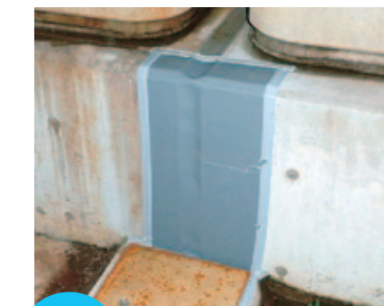
止水 Water stop 高架橋目地止水 Water stop of viaduct joints
